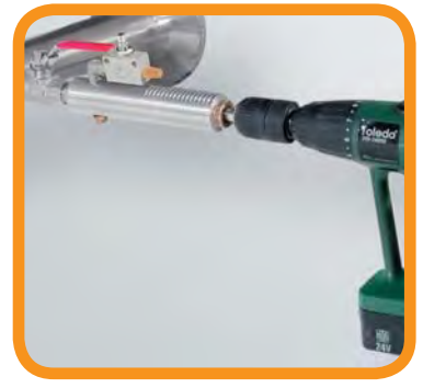
Drilling under pressure with CS drilling jig Order no.: 0530 1108
