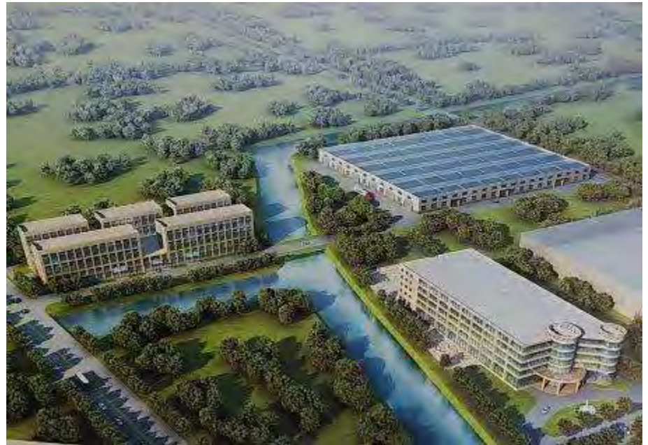
Dynaflox New Factory Buildings
