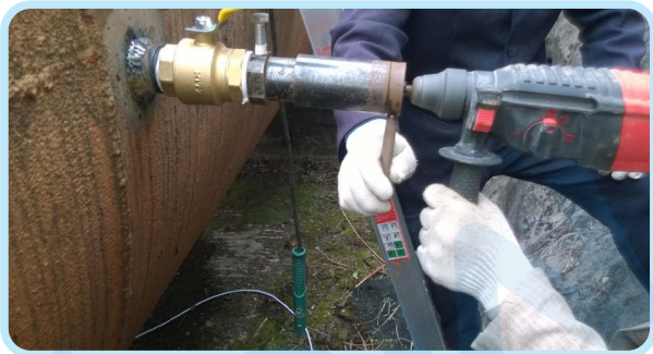
Insertion Transducer Installation
